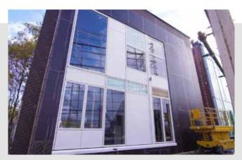
VELFAC offers a CWCT accredited solution. The 62m² large window wall made with 8 complete window units, 20 individual sashes, 6 large opening functions and 5 panel solutions is tested for air permeability, water tightness and wind resistance.
